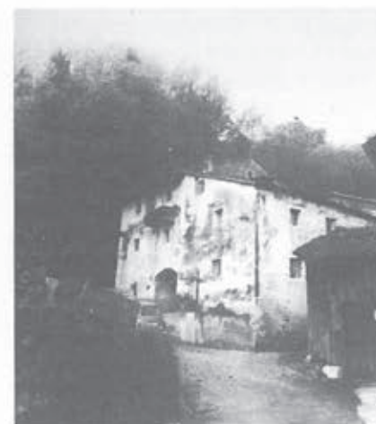
Kraško-vipavski stavbni tip: kmečki dvorec Lisjaki št. 1, 2, 3 The type of the building in the Karst and Vipava, country-seat in Lisjaki 1, 2, 3
