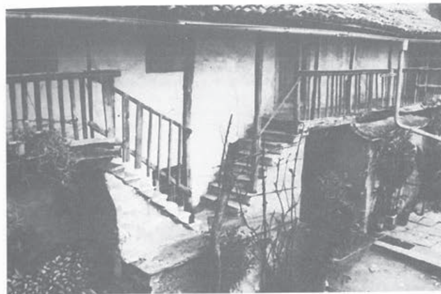
Sl. 4. Kraške hiše v sežanski okolici s tipičnimi ganjki in štengami Pict. 4. A Karst house near Sežana with typical balcon and staircase
